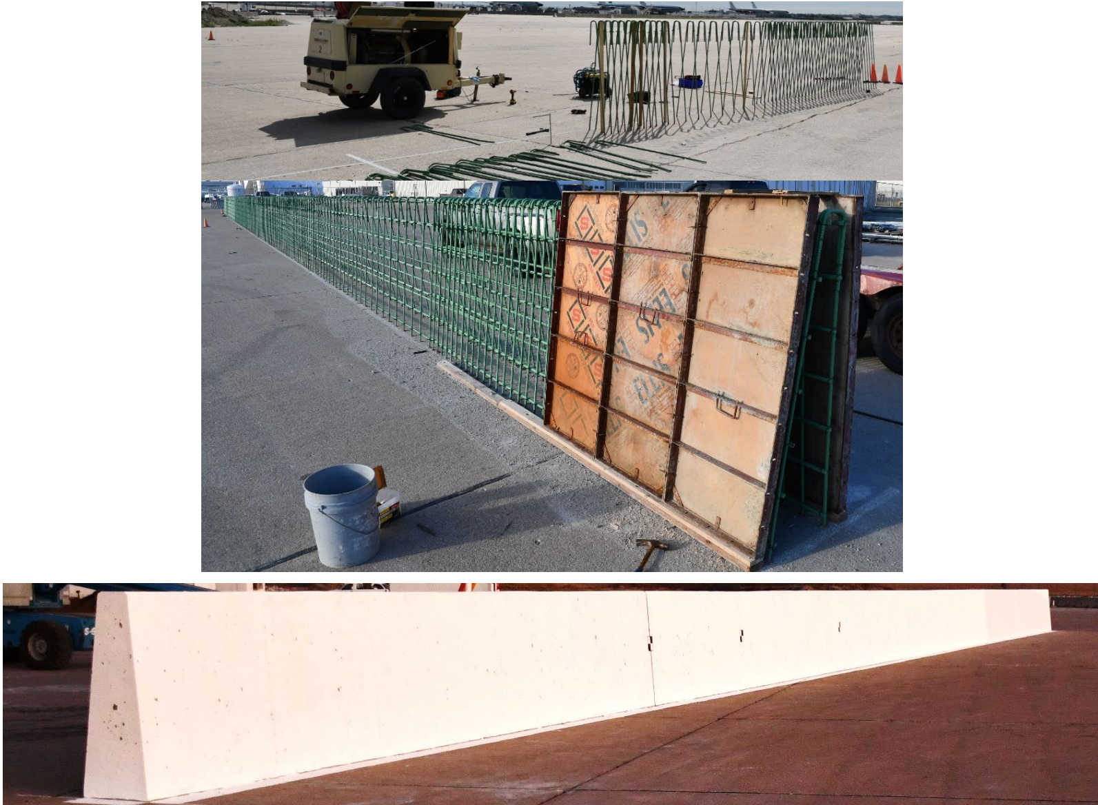
Figure 3.13 Test Article Construction, Test No. MTL6-1
