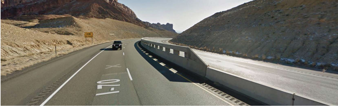
Figure 2.5 Utah DOT 84-in. Tall Roman Wall Installation [3]
